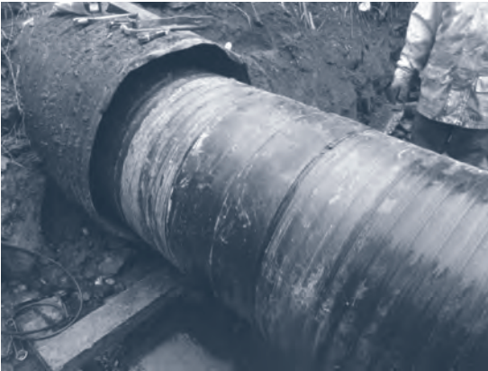
A pipe liner inserted during restoration work at Cheam Lake in 2013.
