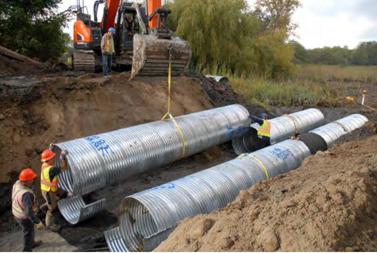
Culvert replacement at 148 Mile Marshes, British Columbia.
