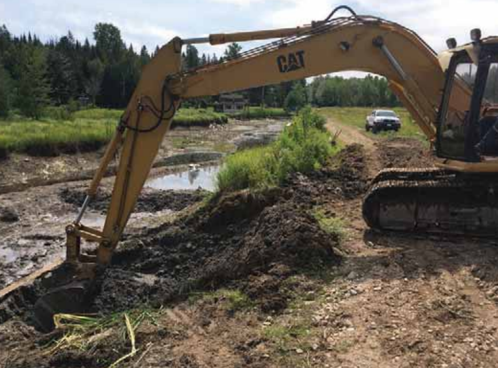
An excavator working at Hazlett's Marsh, New Brunswick.
