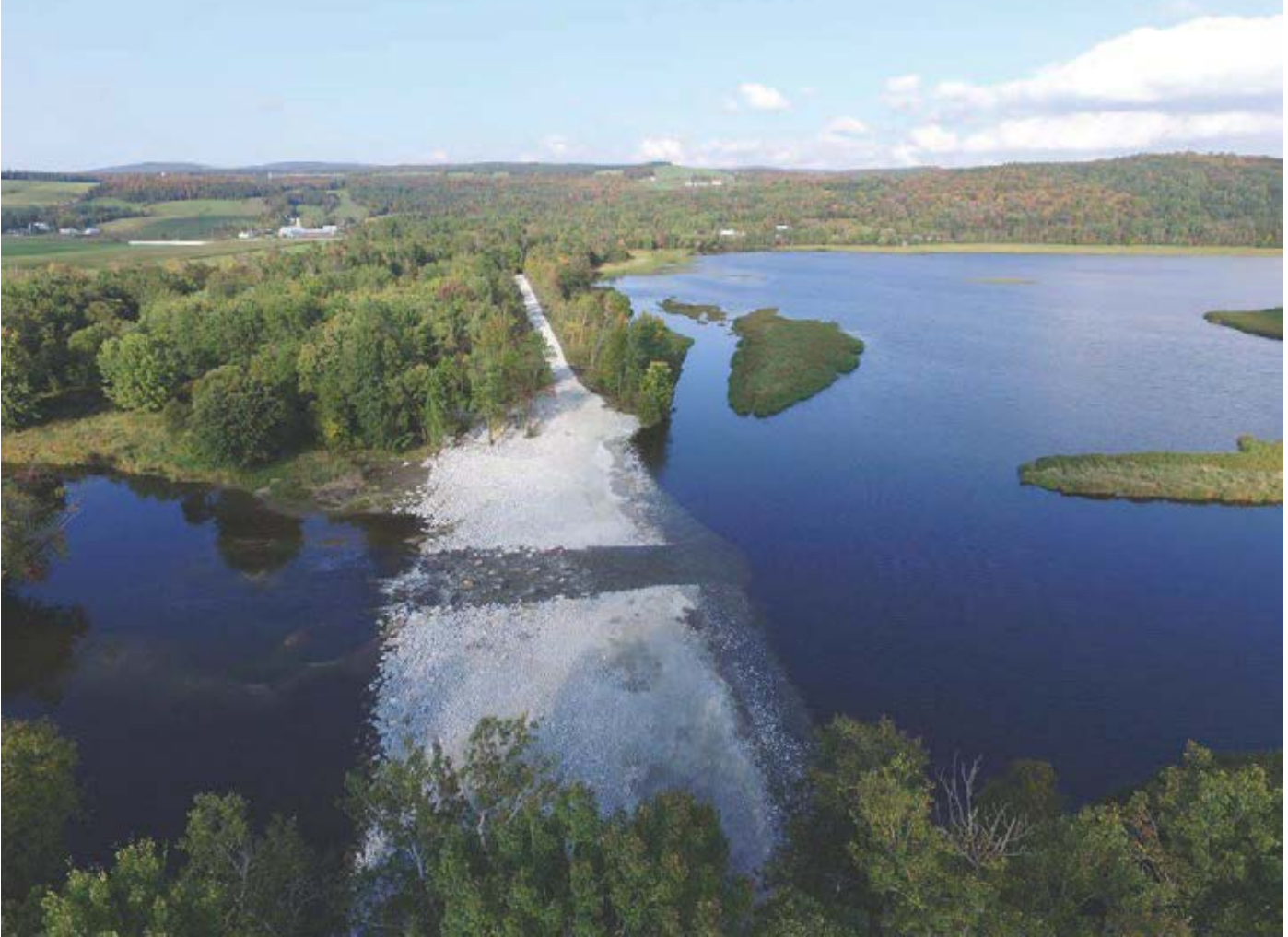
An aerial view of the dam that DUC conservation staff and engineers repaired at the Étang Stater wetland , Quebec.
