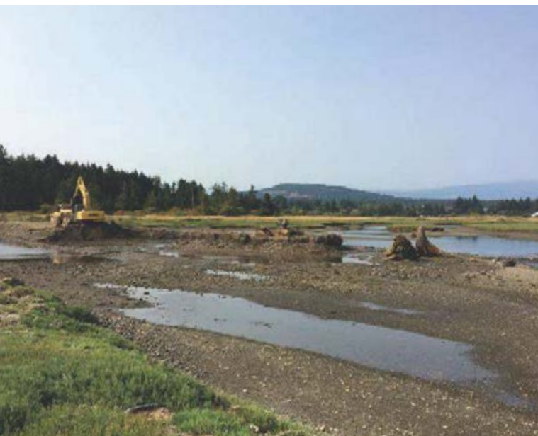
Dike removal at Englishman River estuary, east Vancouver Island, British Columbia.
