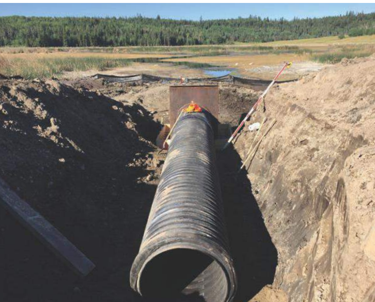
A new water control in place in the Cariboo region, British Columbia, with the wetland in the background.
